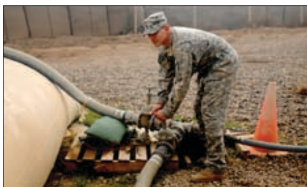
Sgt. Brian Gil, noncommissioned officer in charge of the water site at Contingency Operating Location Poliwoda, Iraq, with the 102nd Quartermaster Company, 80th Ordnance Battalion, 15th Sustainment Brigade, 13th Sustainment Command (Expeditionary), tightens valves leading to the potable water tank Jan. 5 at the COL Poliwoda water site.
